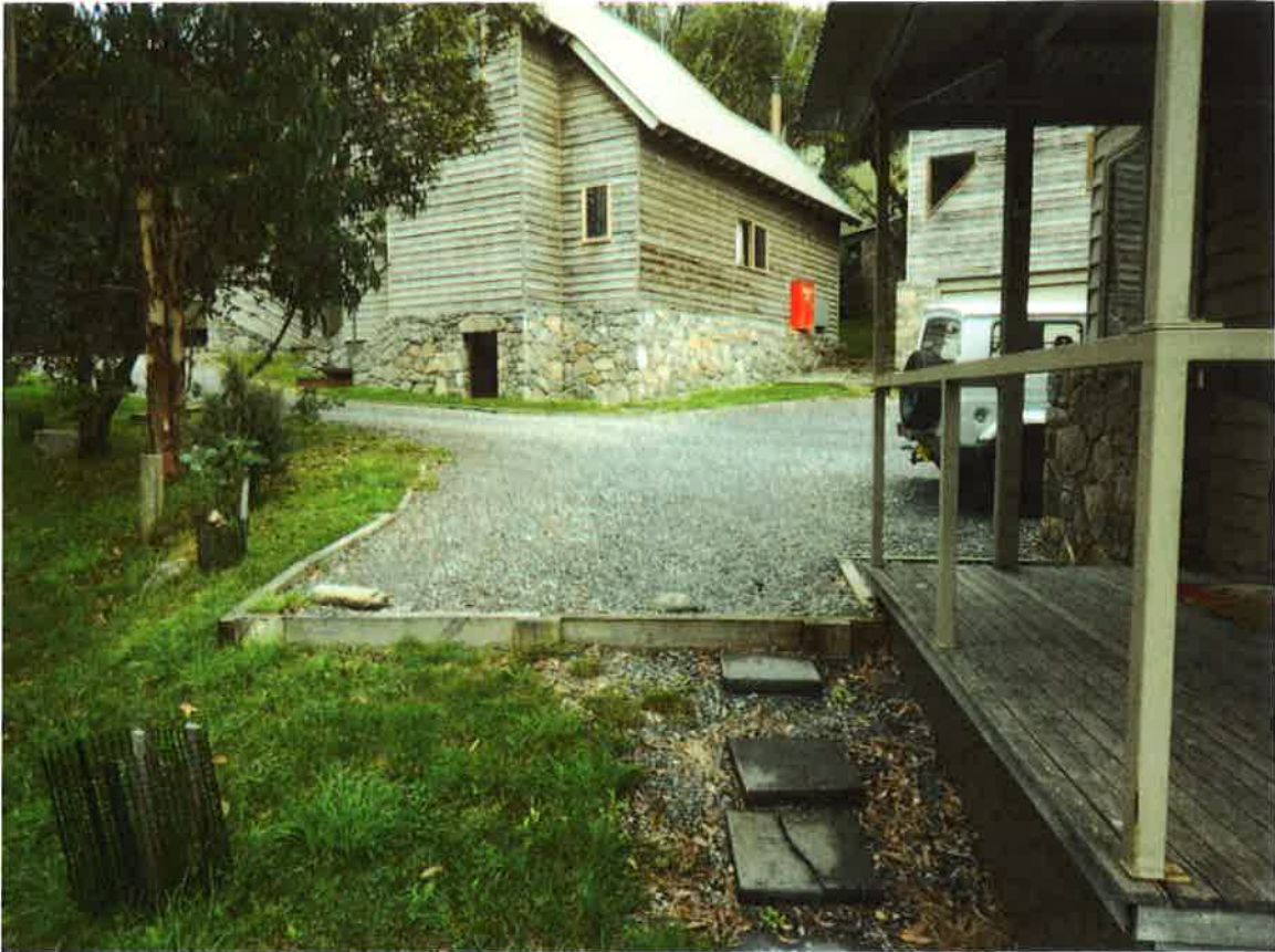
Figure 2: Parking area for construction vehicles
