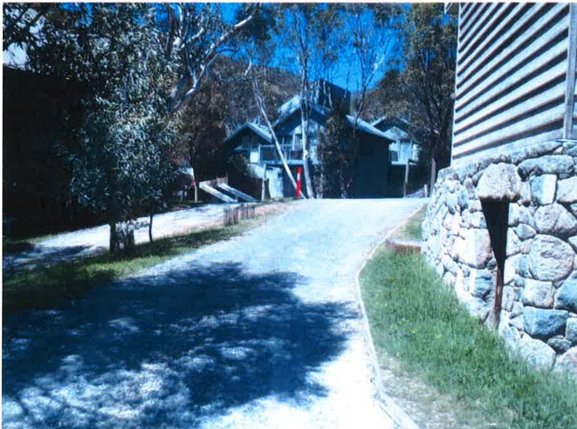
Figure 1: Driveway for construction vehicles
